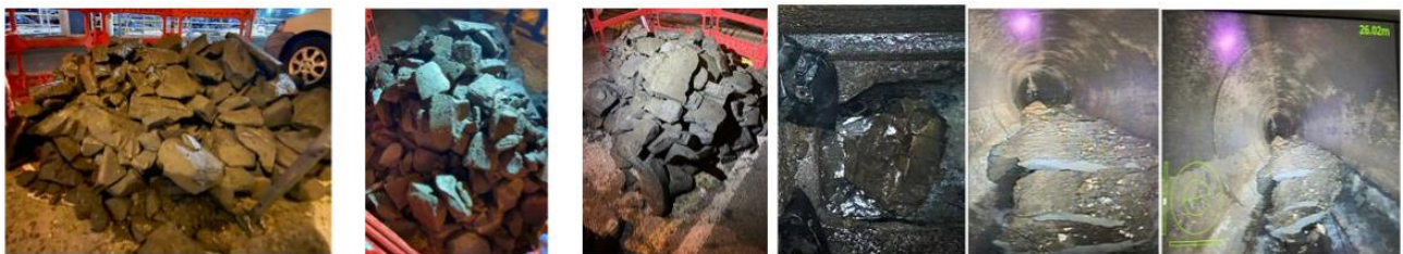
Figure 10: Debris discovered during Ramsgate network capacity survey
