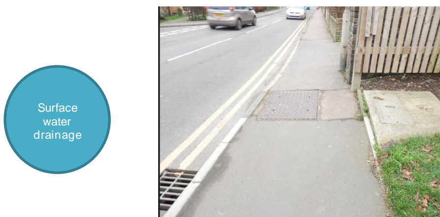
Figure 25 – Existing manhole connection for the Albert Road surface water sewer
