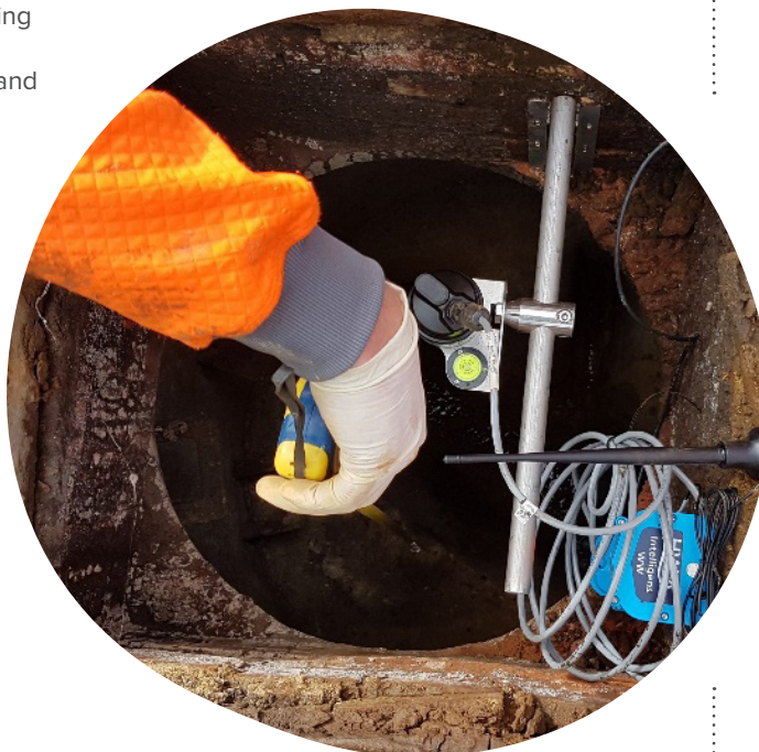
Installing sewer level monitors
