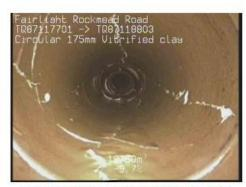
TQ87117701\_Downstream\_231121\_094145\_8297\_63.jpg, 00:03:01, 18.80 m Fractures, multiple at joint from 4 o'clock to 12 o'clock
