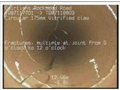
TQ87117701\_Downstream\_231121\_094145\_8297\_60.jpg, 00:01:41, 12.46 m Fractures, multiple at joint from 5 o'clock to 12 o'clock
